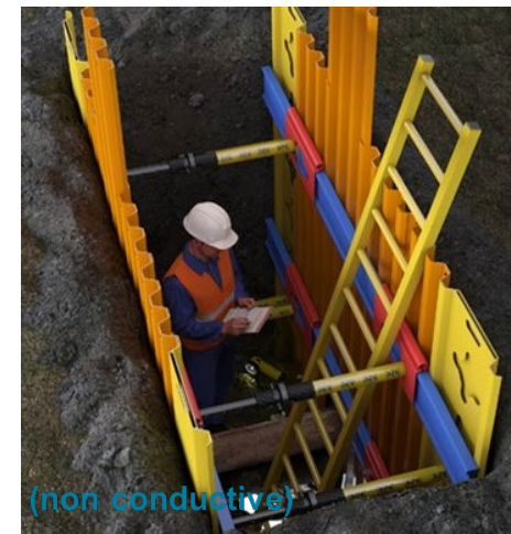
Trench shoring system
