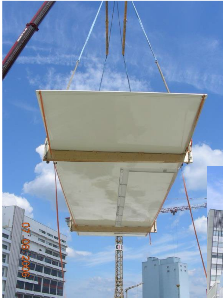
Roof installation on site: simple transport and installation of large-scale elements
