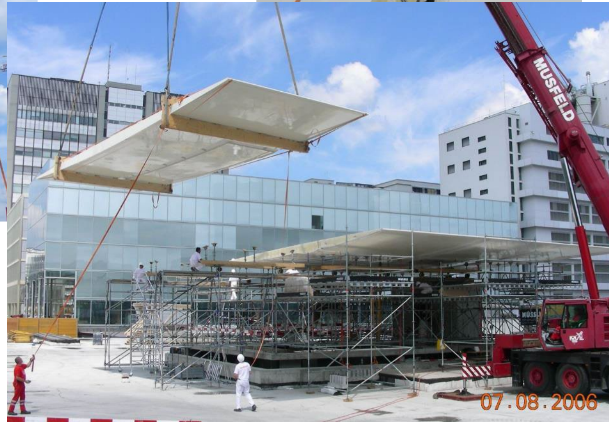
Roof installation on site: simple transport and installation of large-scale elements
