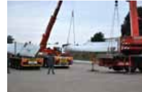
Fig.1 : Unloading of windmill blades at processing site
