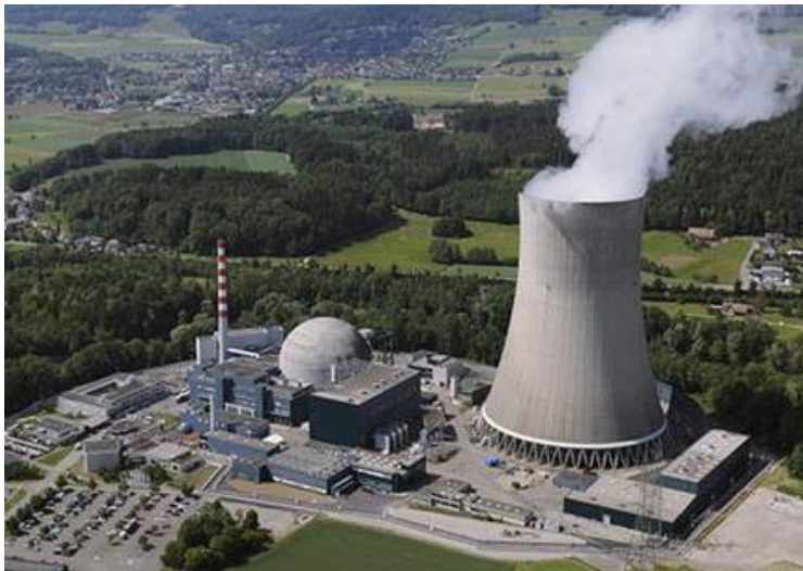
Kernkraftwerk Gösgen-Däniken (KKG) 1060 MW PWR / 40% Net Generation Alpiq 2023: 3218.0 GWh Alpiq is the Managing Partner
