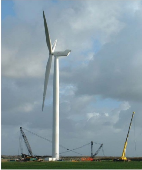
Figure 1 The world's largest wind turbine (summer 2004) at Risø National Laboratory test site, Høvsøre, Denmark. Tower height is 120 m, rotor diameter is 110 m, and generator power is 3.6 MW.
