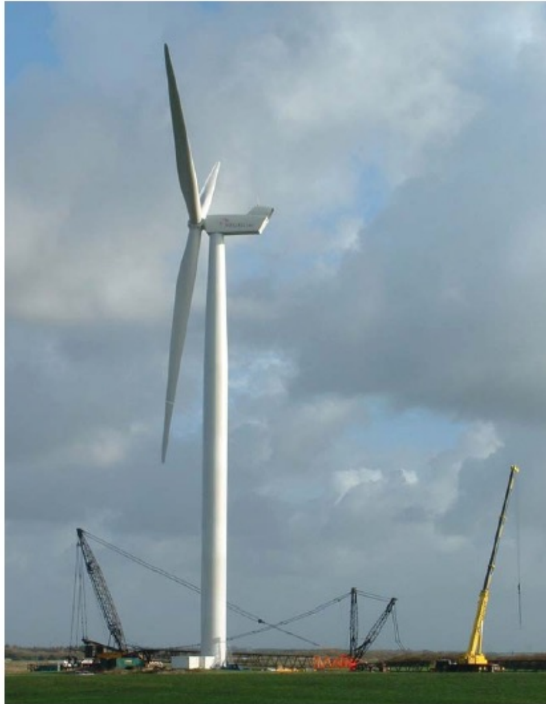
Figure 1 The world's largest wind turbine (summer 2004) at Risø National Laboratory test site, Høvsøre, Denmark. Tower height is 120 m, rotor diameter is 110 m, and generator power is 3.6 MW.
