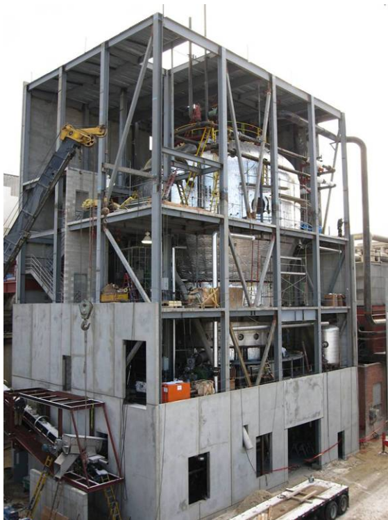
Figure 19. The dryer in Nampa, Idaho under erection.
