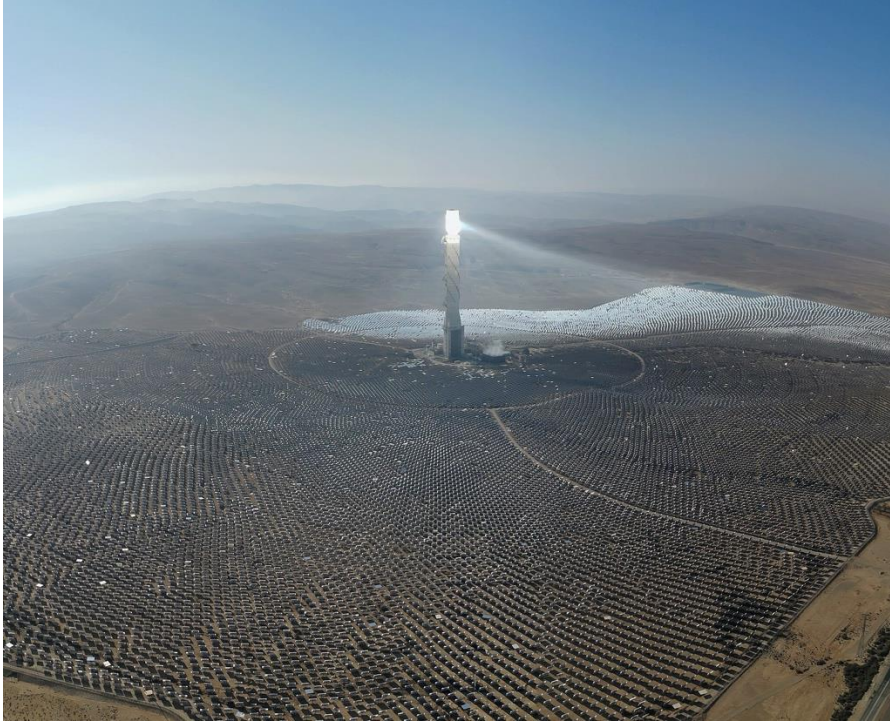
Ashalim Solar Power Station
