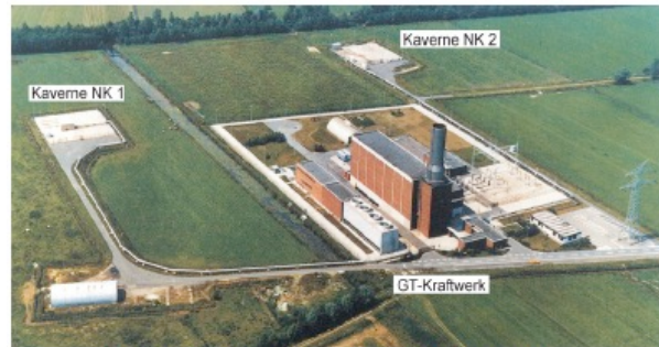
Huntorf (Germany): since 1978, 321 MW e
