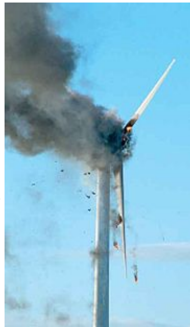
A turbine on fire after an oil leak
