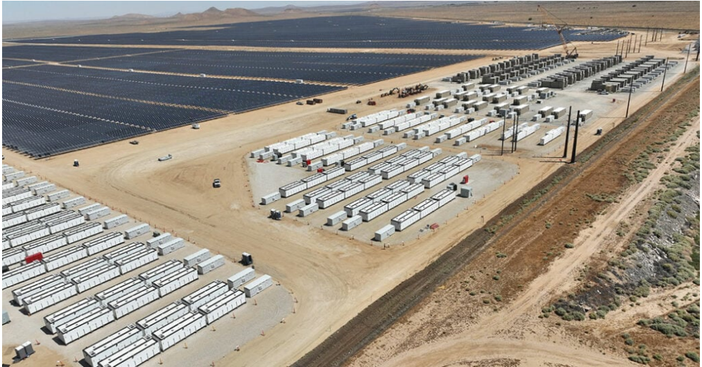
Edwards & Sanborn solar-plus-storage (California, US) 875 MW/3'287 MWh.
