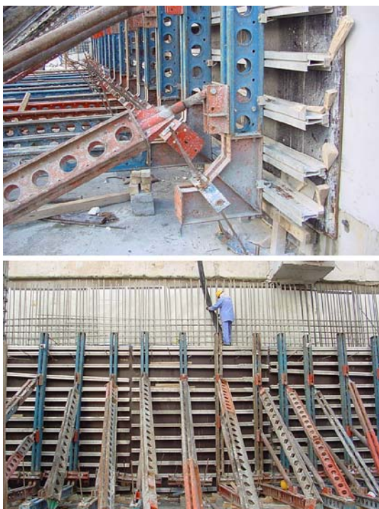
Fig. 8 With self-compacting concrete (SCC) at high casting rates, the formwork should be strengthened especially at the bottom (Courtesy of M Sonebi)
