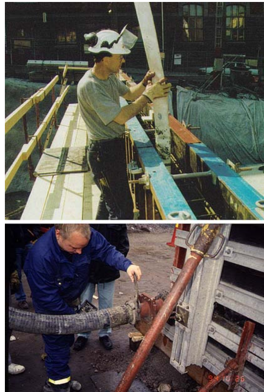
Fig. 11 Casting of wall with two methods (Gravity filling and pressure) (Courtesy of NCC, Sweden)
