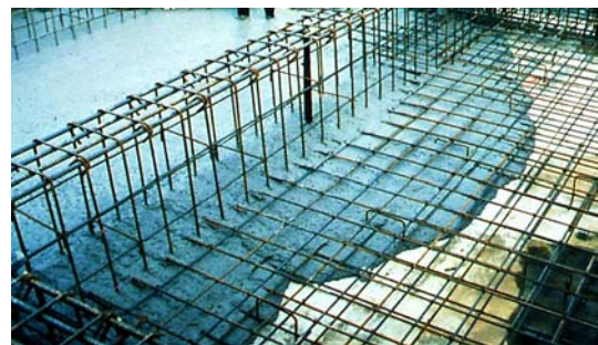
Fig. 2 Self-compacting concrete (SCC) fulfilling requirements on flowability, passing ability and stability
