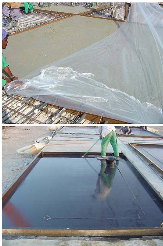
Fig. 12 Good curing practice has to be applied also for self-compacting concrete (SCC) (Courtesy of M. Sonebi)
