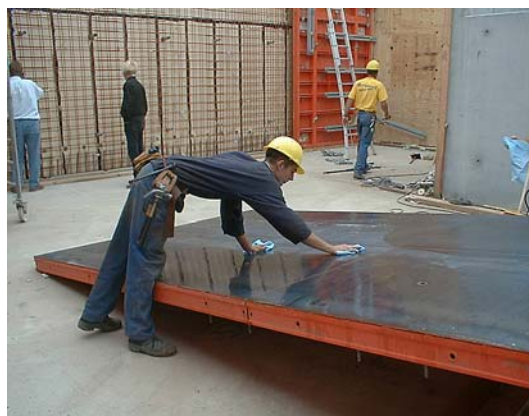
Fig. 10 Properly prepared formwork is important for high surface quality (Courtesy of G. De Schutter)
