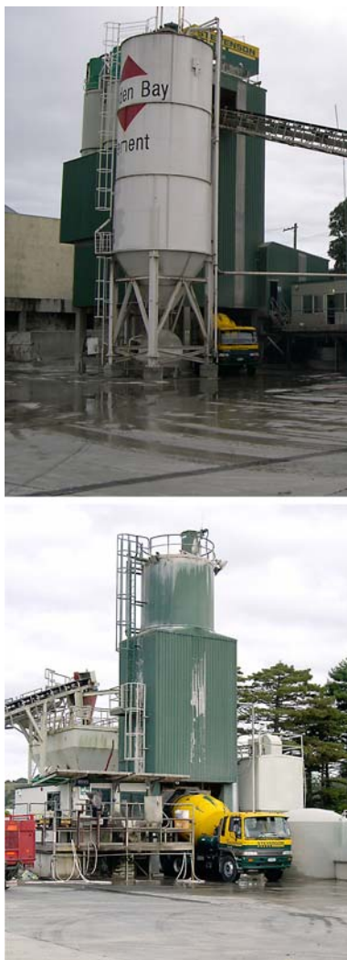
Fig. 6 Both factory mixing and truck mixing is viable for self-compacting concrete (SCC) (Courtesy of M. Khrapko)
