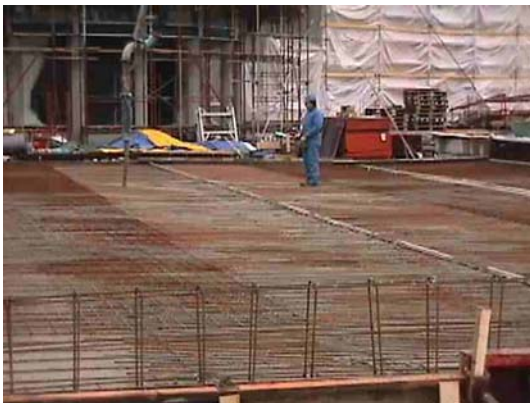
Fig. 1 Casting of self-compacting concrete (SCC) in a one-man operation (Courtesy of NCC Sweden)
