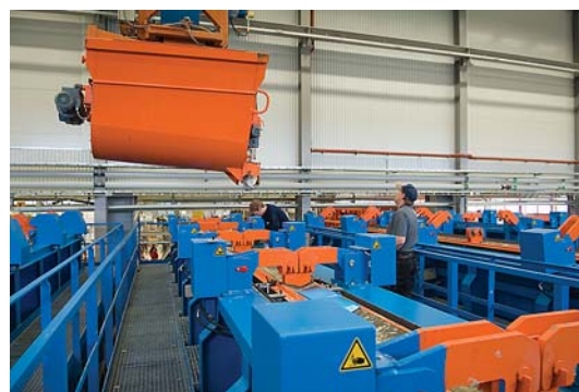
Fig. 13 Walls being cast with self-compacting concrete (SCC) as an integrated part of the fully industrialised prefabricating house building system NCC complete (Courtesy of NCC, Sweden)
