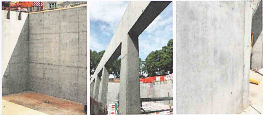
Figure 10.5 Construction of multipurpose sports facility at Uranienborg, Oslo, Norway. Left: Newly cast walls. Mid: Columns and beams. Right: Achieved surface quality.
