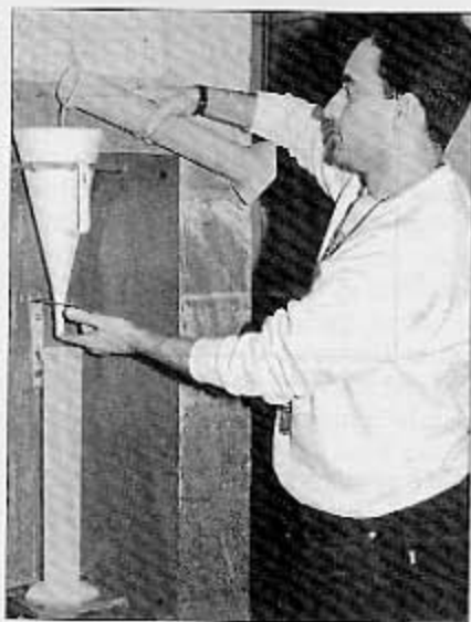
Fig. 5 — The Marsh cone test.
