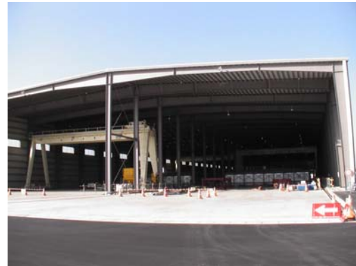
Photo 4 UFC slab factory
