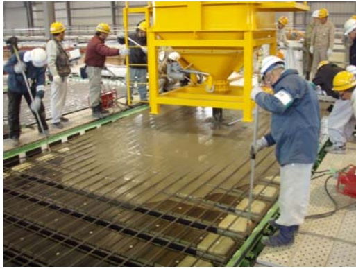
Photo 6 Pouring UFC to slab
