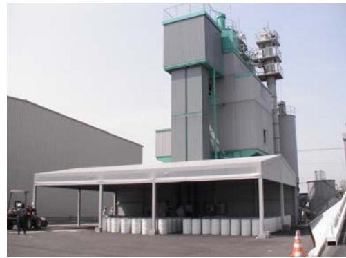
Photo 3 UFC batching plant
