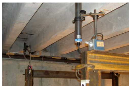
Photo 2 Measuring displacement of slab
