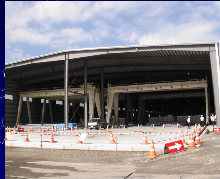
Ductal slab production factory
