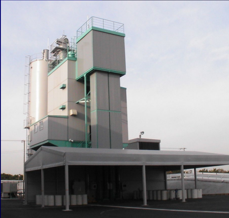
Ductal Batching Plant
