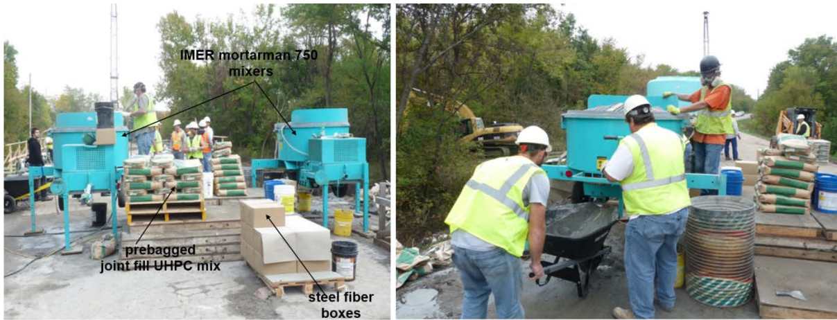
Figure 81. Photos. Batching of UHPC joint fill using IMER Mortarman 750 mixers in field.
