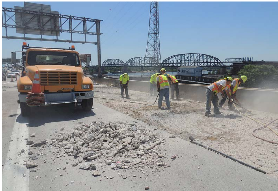
Figure 67. Photo. Jackhammering deck sections prior to removal.
