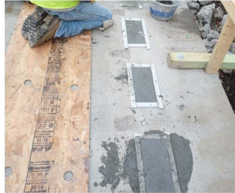
c) Shear pocket with UHPC joint fill
