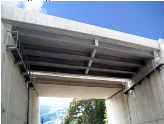
Photo 11 Horikoshi C Ramp Bridge
