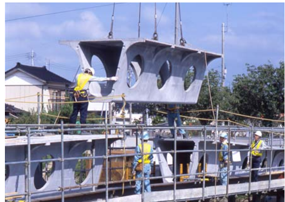
Photo 2 Erection of center block
