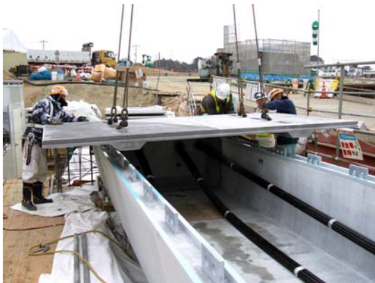
Photo 14 Setting UFC slab (thickness 7cm)
