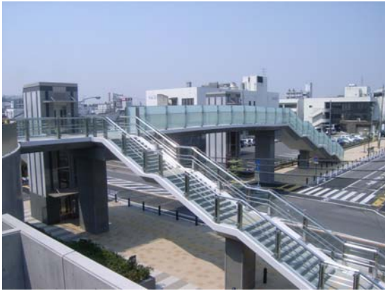
Photo 4 Toyota City Gymnasium Footbridge
