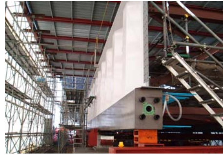
Photo 12 UFC lower beam with corrugated steel web
