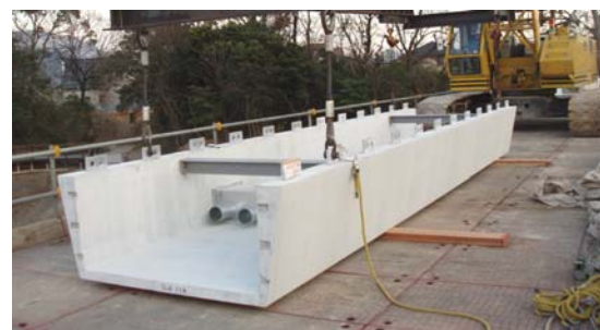
Photo 13 Precast block of Mikakeike Bridge (width:2.1m, length: 10.5m, weight: 9.2t)
