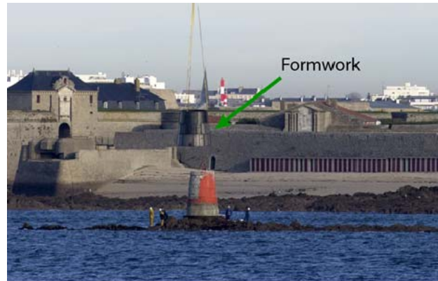
Installation of formwork
