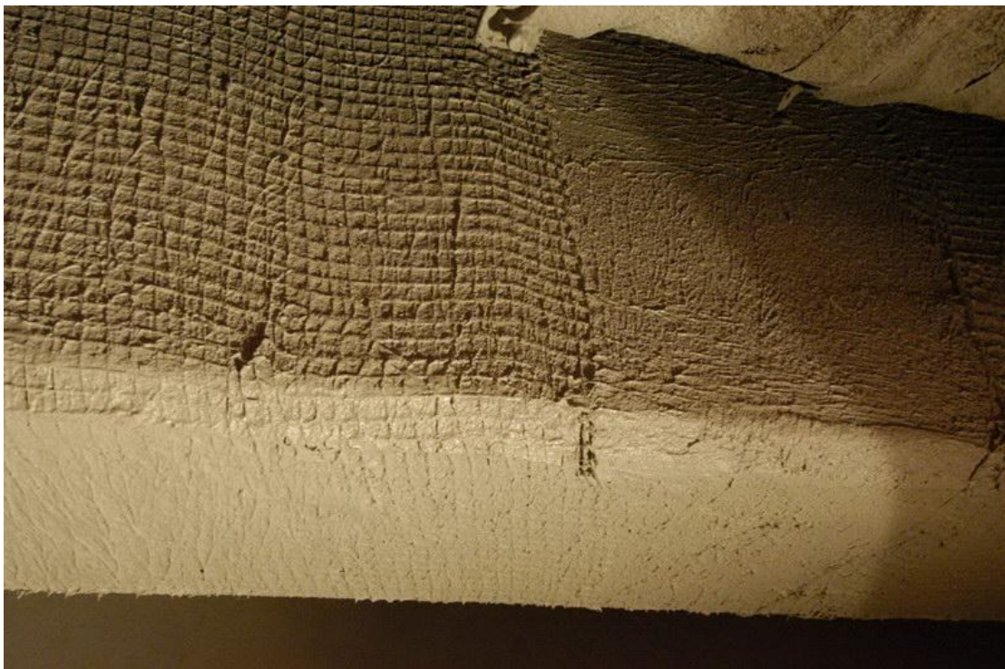
Figure 8 Carbon fibre mesh applied in first layer of cementitious mortar (to be finished with another layer of mortar)
