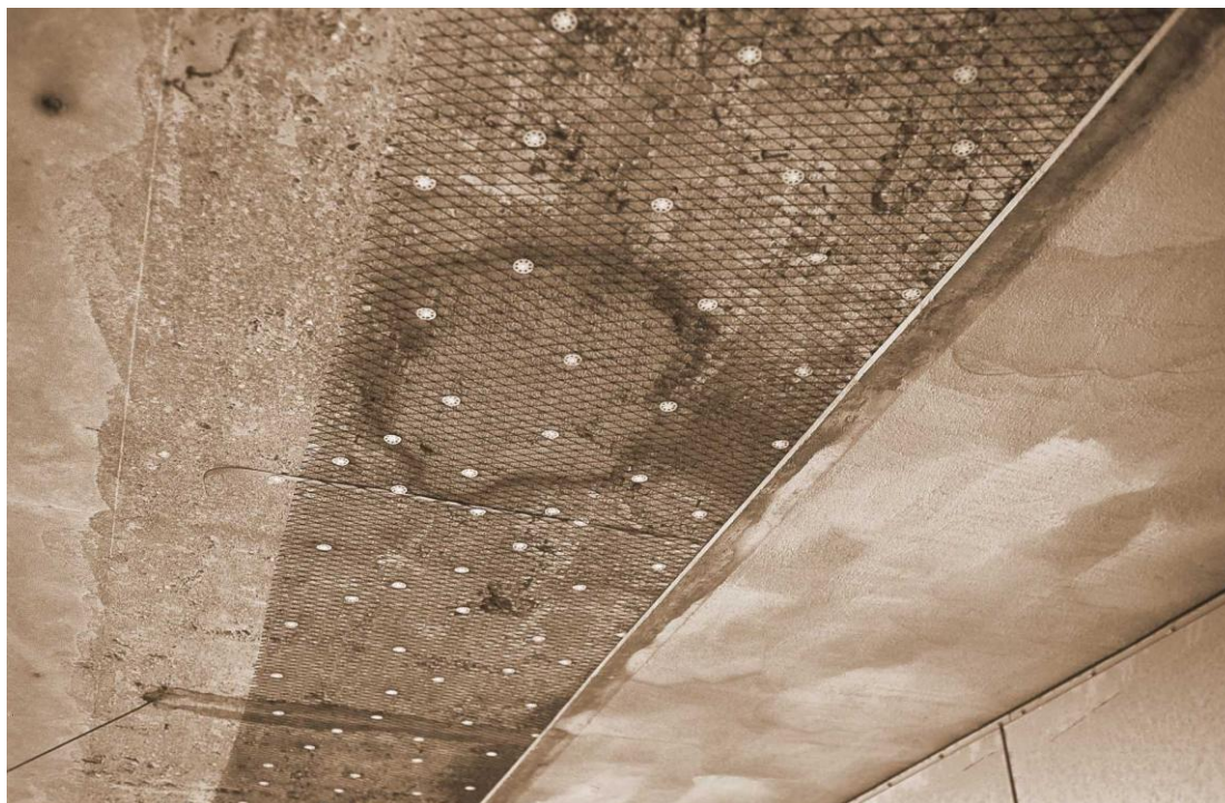
Figure 6 Three stages of application of a titanium mesh to the underside of a concrete slab; left : prepared surface; middle : titanium mesh attached (note repair patch and plastic fixing pins); right : shotcrete overlay applied
