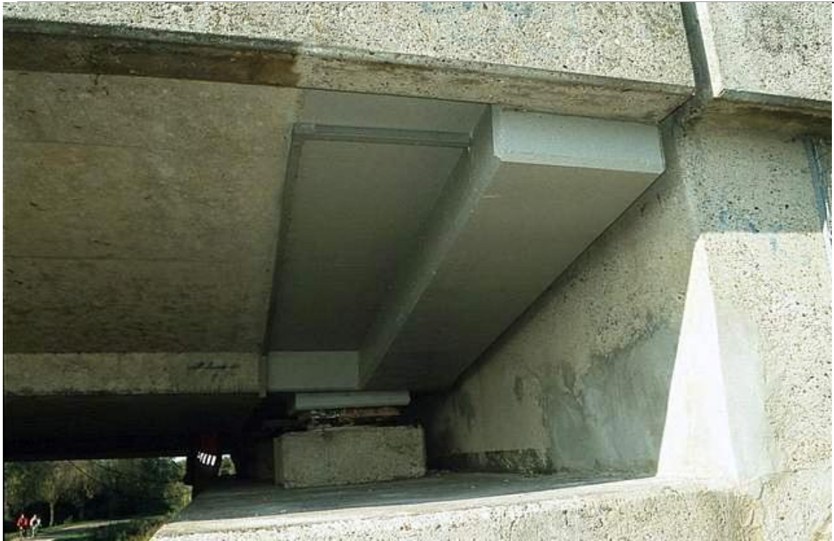
Figure 7 Conductive coating anode applied on edge beam of bridge deck adjacent to abutment
