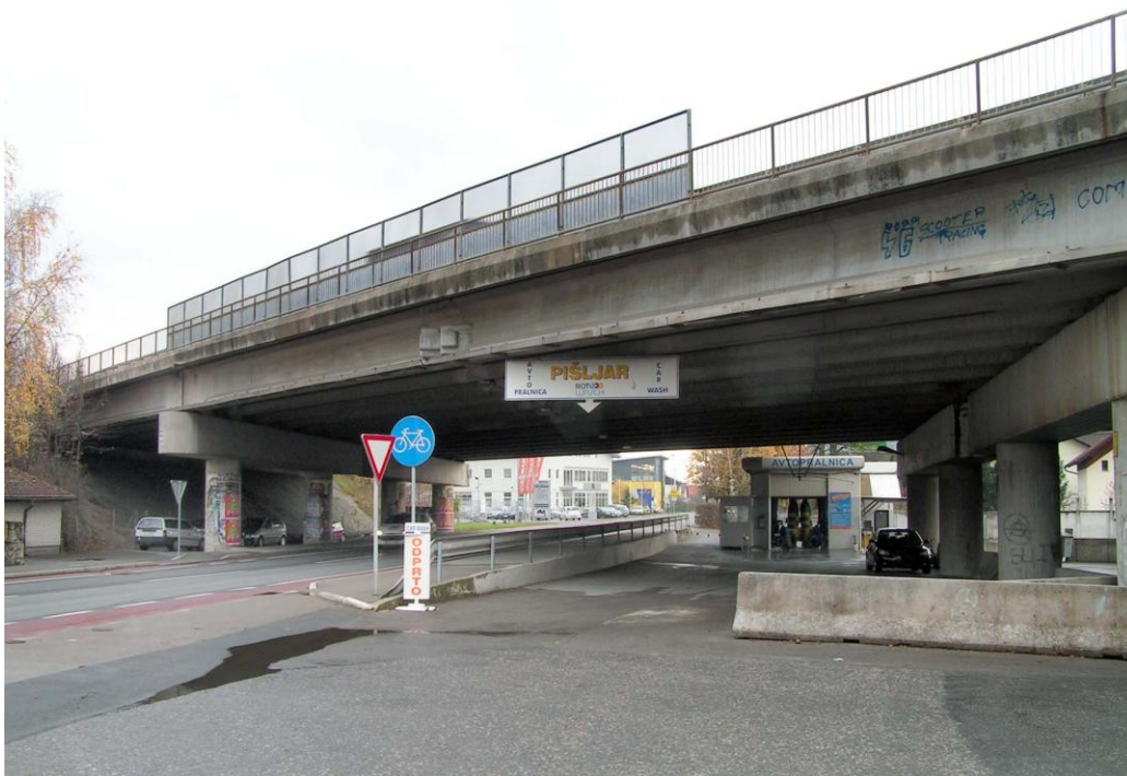
Figure B.4 Overpass view from NE
