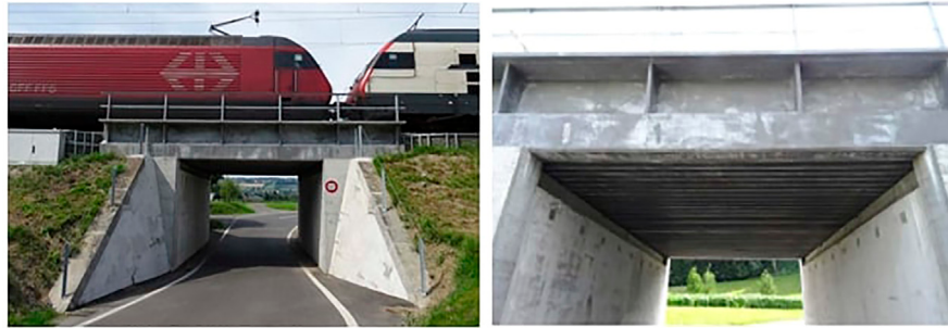
FIGURE 13 | Railway underpass Unterwalden (Sempach) with a structure in R-UHPFRC resting on concrete abutments. (Photographs: E. Brühwiler).
