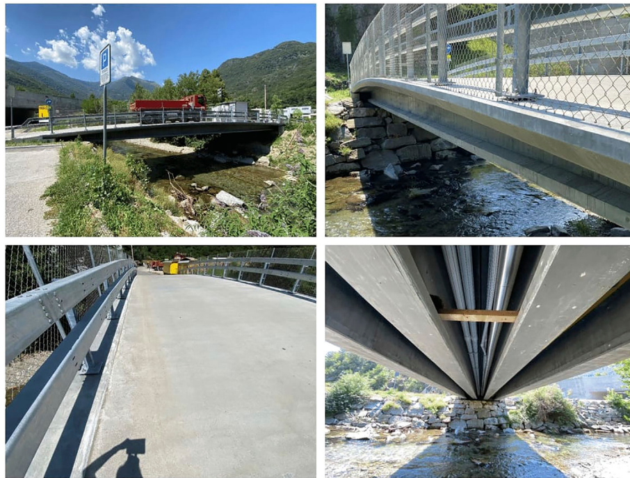
FIGURE 14 | Taverne bridge. (Photographs: E. Brühwiler).
