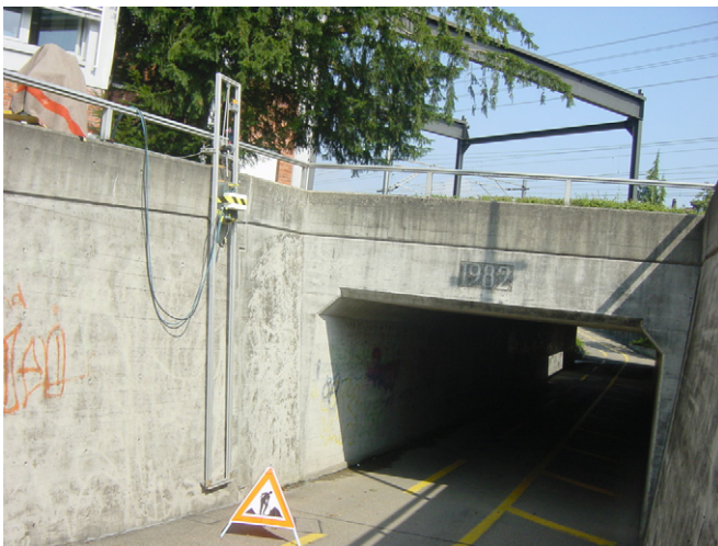
Fig. 1. Retaining wall with acquisition apparatus.
