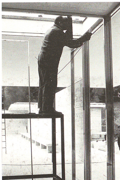
Fig. 73. Positioning the windows in their stainless steel frames.
