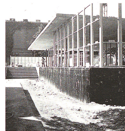
Fig. 70. The structure of the podium and the concrete roof before being clad with stone.
