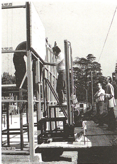
Fig. 61. The process of positioning the travertine slabs.
