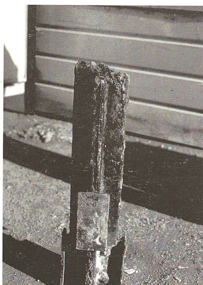
Fig. 51. Discovery of the foundations of the 1929 Pavilion. The anchoring of a metal pillar.
