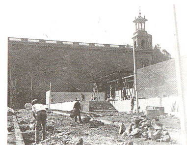
Fig. 22. The metal structure of the roof during construction.
