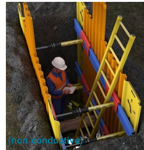
Trench shoring system
