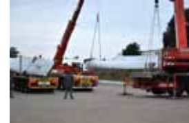
Fig.1 : Unloading of windmill blades at processing site
