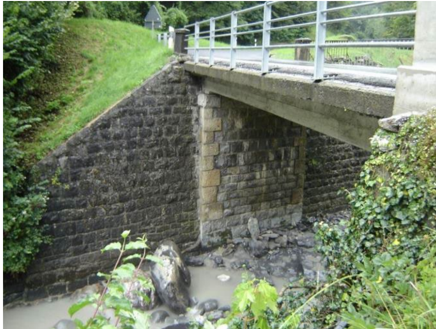
Old one-lane bridge
