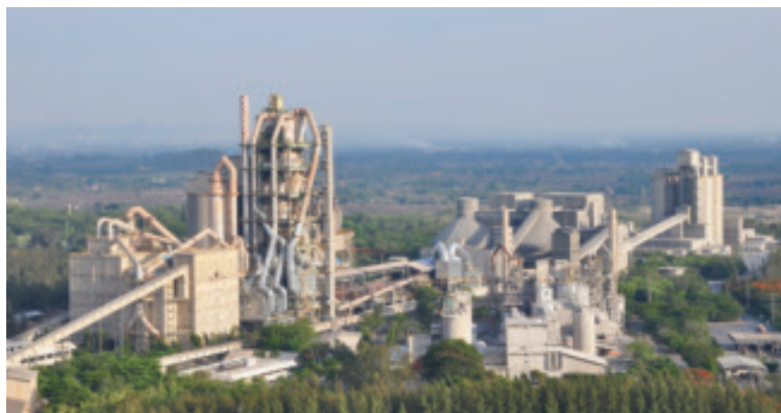
The disposal of composite waste in cement kilns is widely believed to be an effective option, resulting in energy and materials recovery. (Picture used under license from Shutterstock.com © Parnumas Na Phatthalung.)
