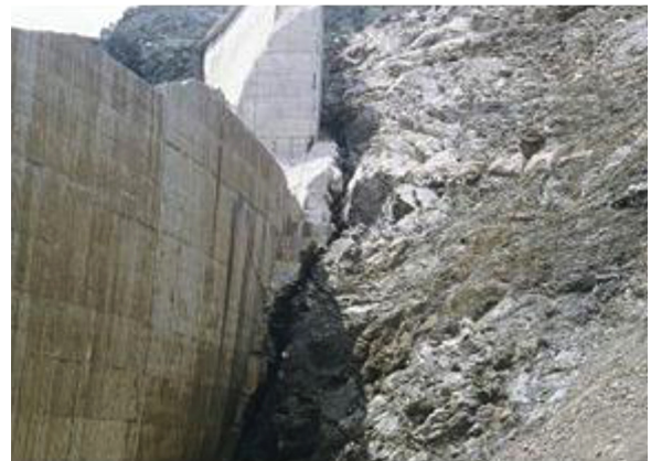
Fig. 5. The most conspicuous features of the site exposed after failure. Top, the “dihedral” excavation with half of the thrust block fallen after the flow (the exploratory adit at right was bored early after the failure to make jack tests in situ); below, a wide crevice is open just upstream of the concrete arch, wider at the base and closing more higher (photos Duffaut, 1960).
