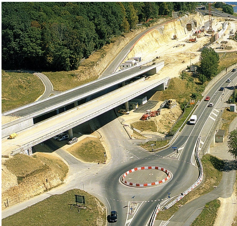
Roads and transportation structures
