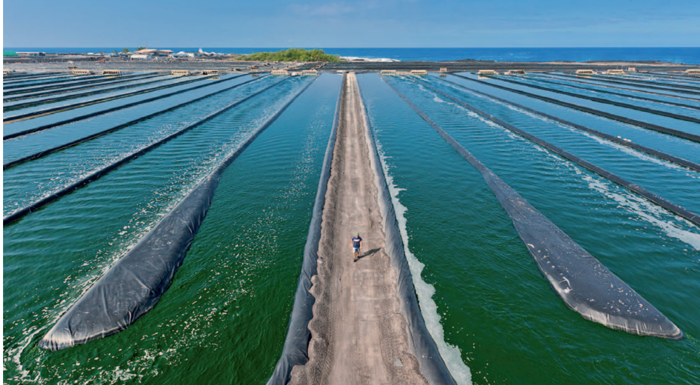
Algae farms require vast water surface areas to efficiently convert sunlight into an oil used as a biofuel.
